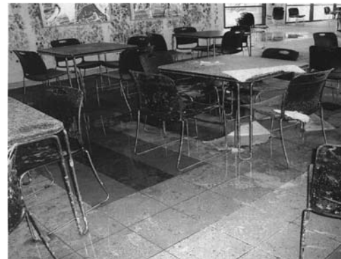
The flooded cafeteria at Xavier University, which had to be replaced due to mold. Photo by Irving Johnson III and Marion Bracy.
